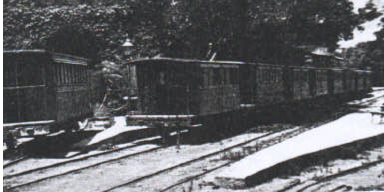
First and third class train stationary in Hamrun station; headquarters and workshops on left
